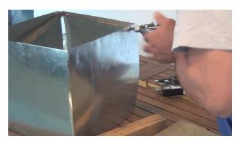
The aluminum rivets can be flattened using the hammer.
