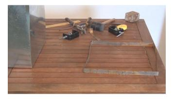
I drill 5mm holes to insert popping rivets securing the steel ribbon to the steel cube.
