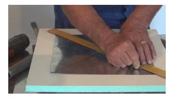
The hose should come through the layers of bitumen and steel wool as well. So I measure and mark the center of the bitumen pieces and drill the hole.
