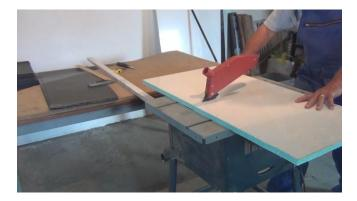
I will cut some wood pieces 2 x 2 x 16 inches which I will use to secure the EPS in place with screws.
